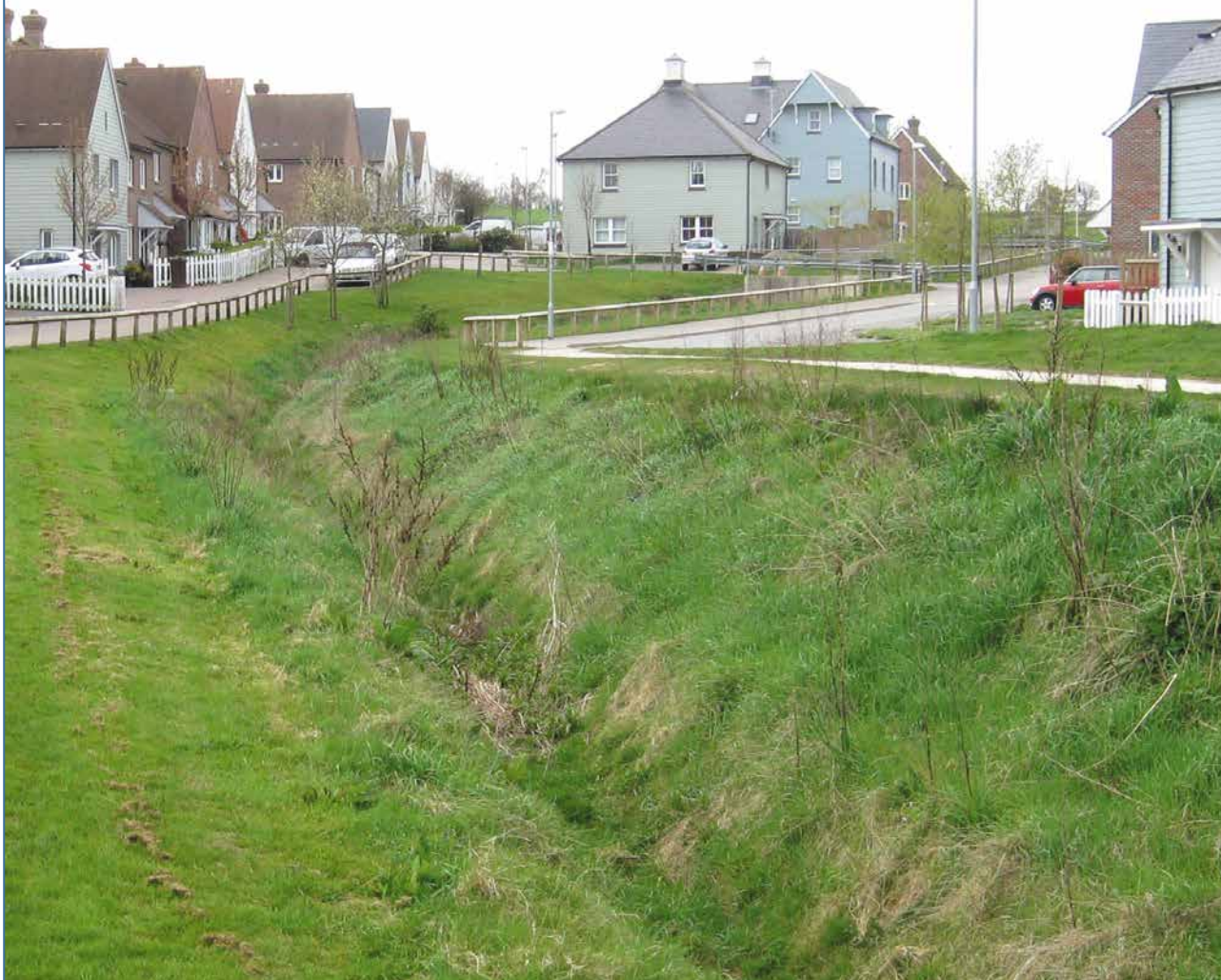
Swale at Valley Park, Rye, East Sussex (Source: Richard Wilson, Rother District Council)
